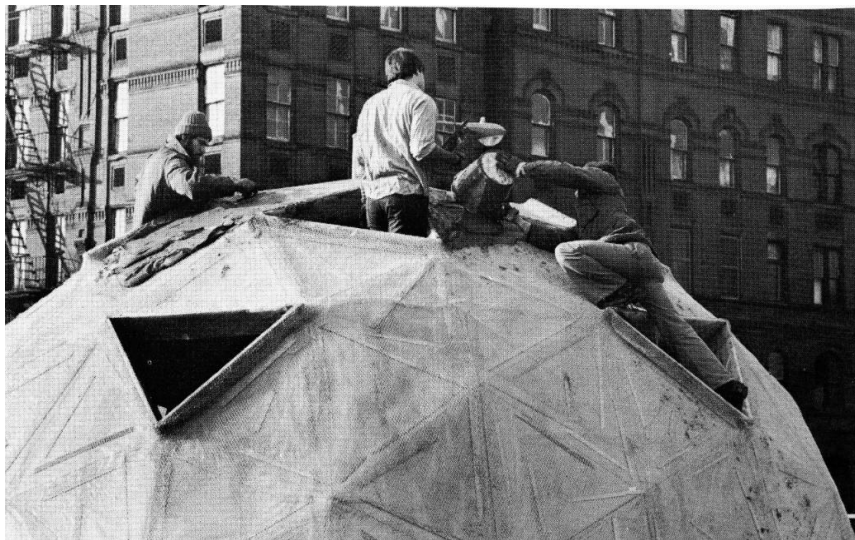
Fig. 3.1; CHARAS members work to add cement coating to a full scale geodesic dome.
