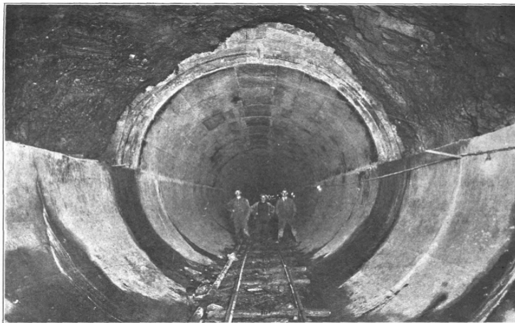
Rondout Pressure Tunnel, 14½ feet in diameter, typical of other pressure tunnel work
