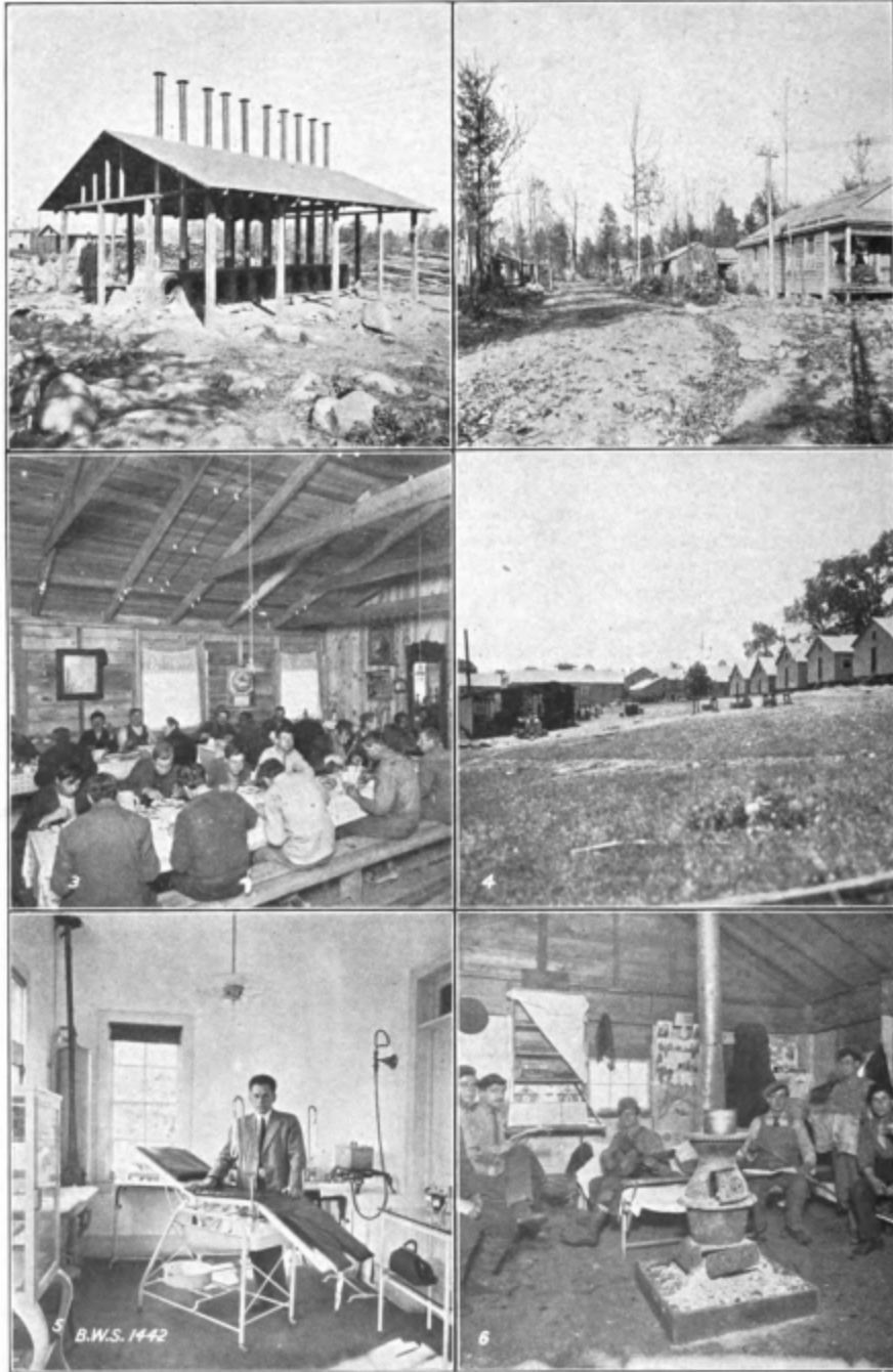
CONTRACTORS' CAMPS—(1) Outdoor stoves at Camp Hill View. (2) Chadwick avenue at "Camp City" at Ashokan. (3) Mess hall, Camp Hill View. (4) Camp Blakeslee near Croton lake, now completely obliterated. (5) Operating room in contractors' hospital. (6) Recreation at close of legal 8-hour day.
